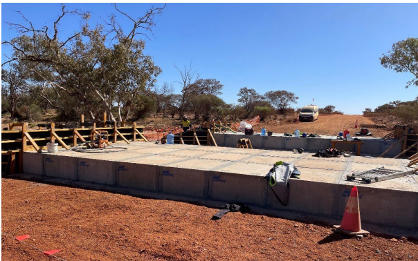
Figure 13: Jones Creek Crossing site works underway
