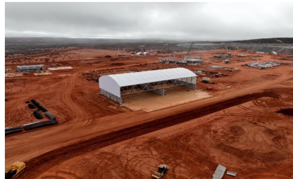
Figure 8: Concentrate storage shed
