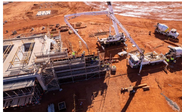
Figure 6: Concrete pour at the fine ore bin
