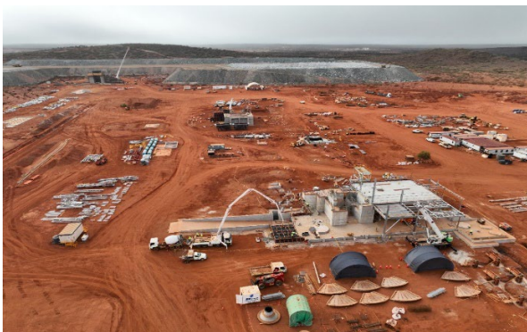
Figure 5: Process plant construction
