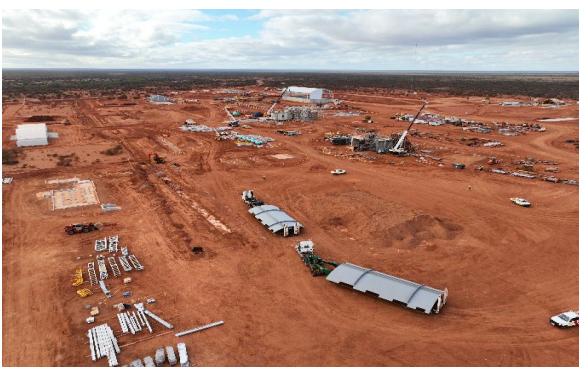
Figure 7: Fine ore bin segments arriving on site
