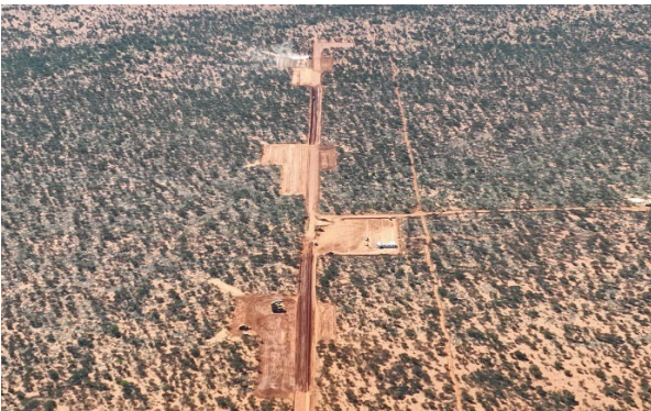
Figure 11: Earthworks for wind turbines
