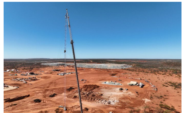
Figure 12: 90-metre-high communications mast being erected
