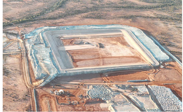
Figure 2: Tailings Storage Facility 1
