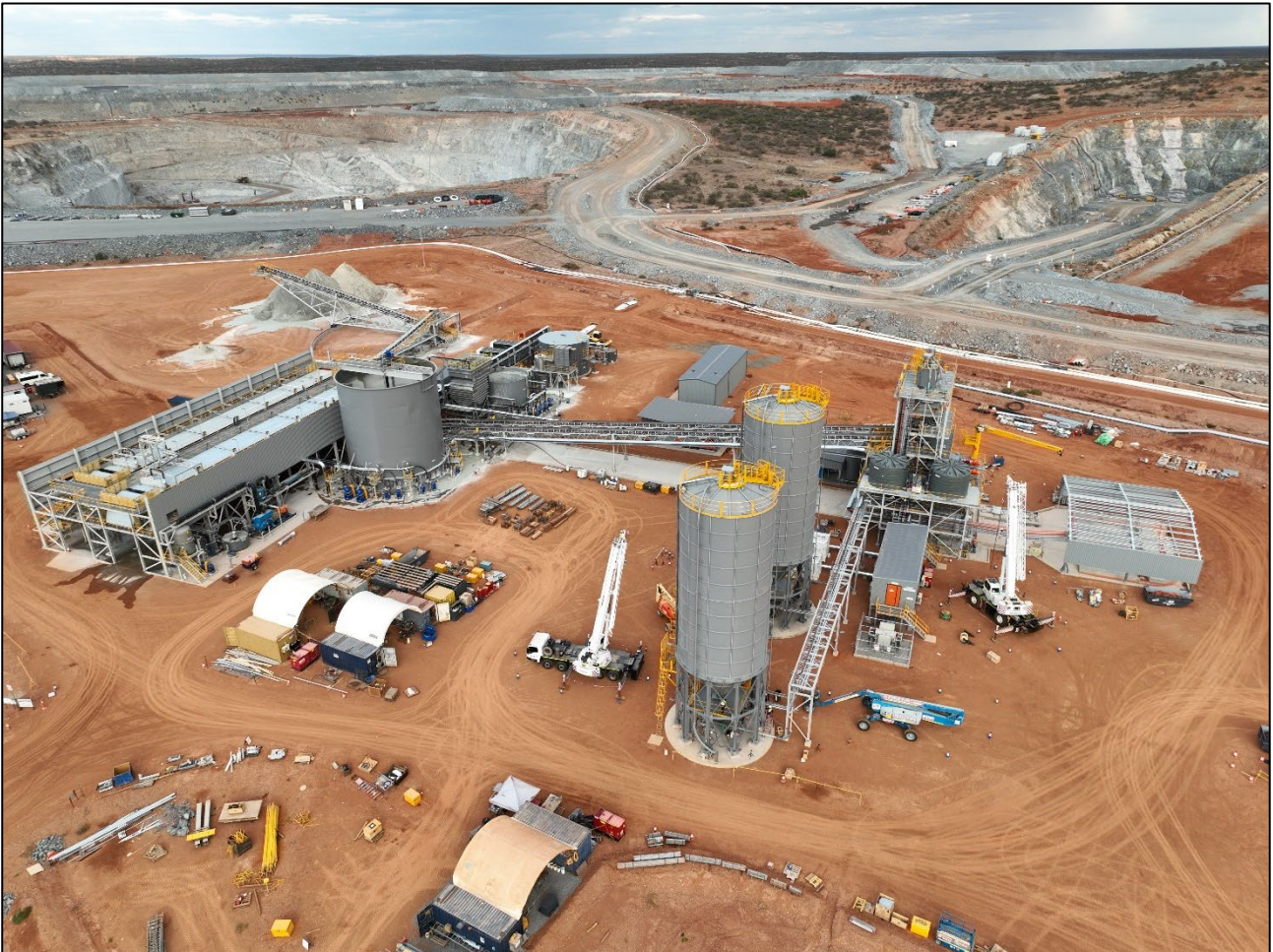
Figure 13: Aerial view of the paste plant
