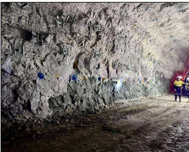
Figure 3: Underground mining operations
