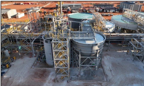
Figure 9: Water storage, thickening and concentrate settling
