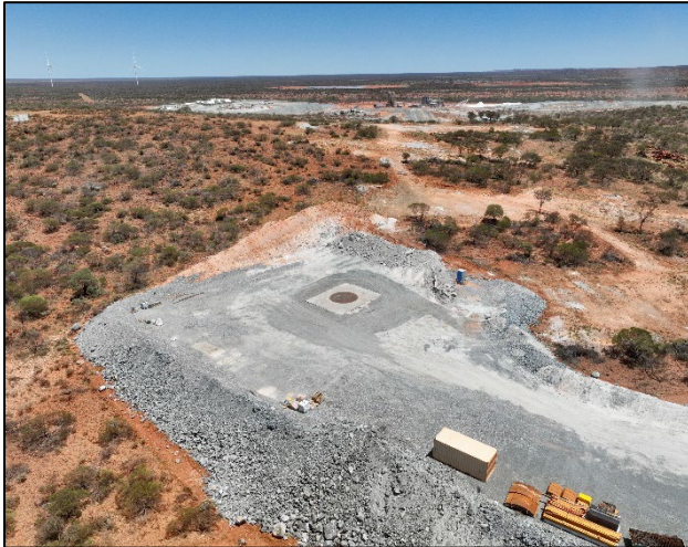
Figure 3: Southern ventilation raise bore site ready for raiseboring activities
