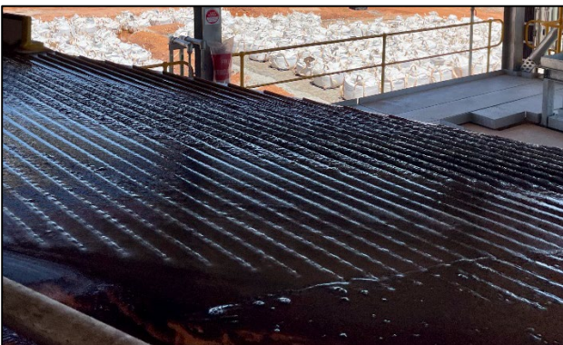
Figure 9: The tantalum circuit in operation
