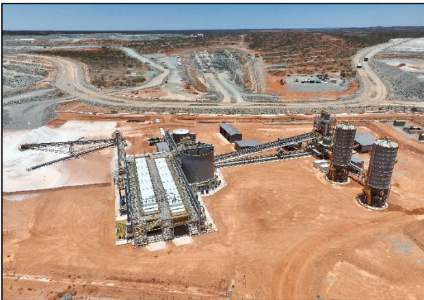
Figure 13: The completed 4Mtpa paste plant
