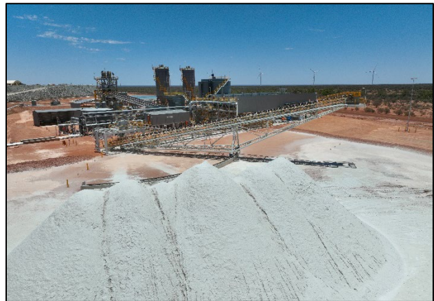
Figure 14: Dry stacking tailings from the paste plant
