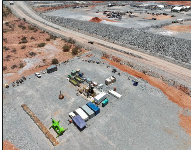
Figure 4: Northern ventilation raise bore site – Drilling in progress
