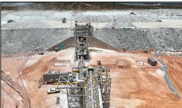
Figure 7: Primary crushing in operation
